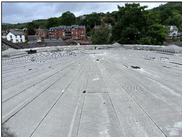
Figure 3: The roof of the building.
